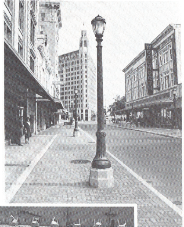
10cm Hollandstone pavers were used in construction of streets.
