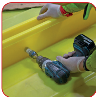
Step 4 Once drilled, proceed to drill the same holes using the 27mm hole saw
