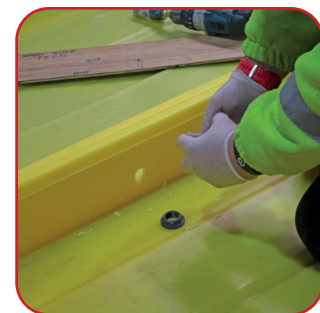
Step 6 Unscrew the nut from the BFC connector (left-handed thread)
