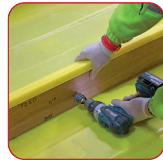
Step 3 Measure on the inside, from the left-hand side, 410mm from the inside edge, and 42mm up from the base. Once marked, begin drilling
