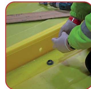
Step 6 Unscrew the nut from the BFC connector (left-handed thread)
