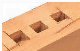
Drill Square Holes
