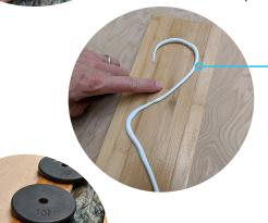
Squeeze out a bead of silicone about a 1/8" thick. Curve it around so that the whole board will be secured to the plywood.
