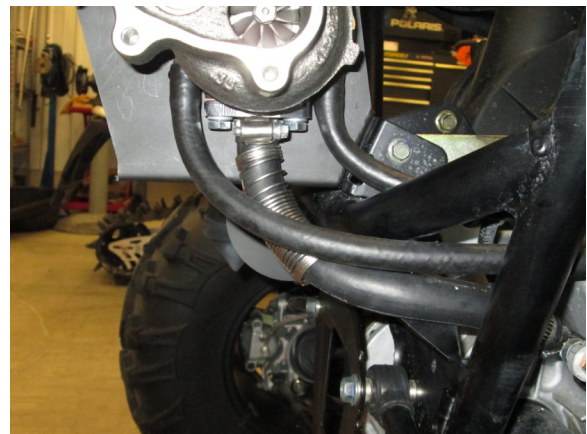
24. INSTALLING OIL DRAIN LINE Locate the oil drain line and fasten the 5/8" side of the hose to the turbo oil drain using a #12 hose clamp.
