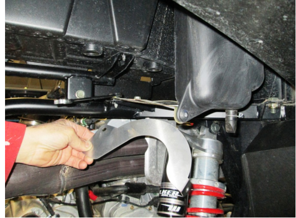
38. INSTALL MUFFLER Remove the bed support bracket on the passenger side of the vehicle.
