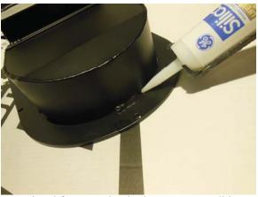
5. Optional for operation in deep water conditions (submersion in 12" or more), silicone between the welds on both clutch covers using weather proof silicone.
