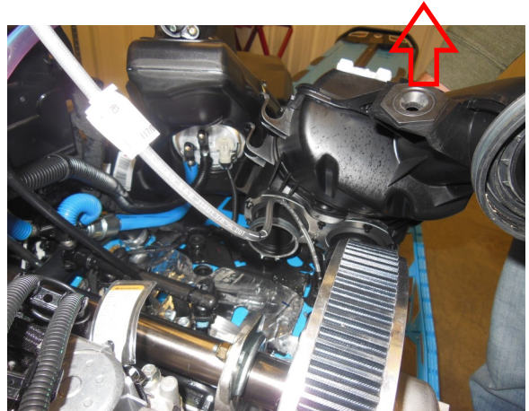
28. Lifting from the bottom, remove the factory air-box. Make sure hoses/harnesses are free
