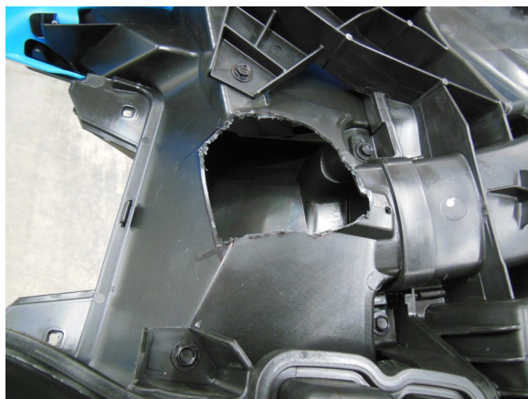
95. Mark intake ducting as shown on template and carefully cut
