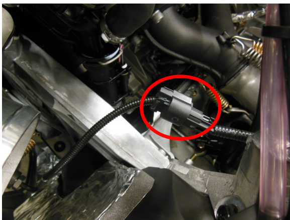
63. Install muffler temp-sensor connection and tighten sensor-nut on muffler
