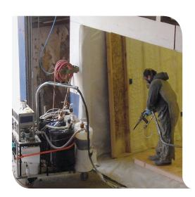
While the chemicals that make up two-part foams and coatings are safe and nontoxic once mixed together, the base chemicals are hazardous for workers. Base chemicals are packaged in closed-system bulk containers with preinstalled single-use dip-tube assemblies.
