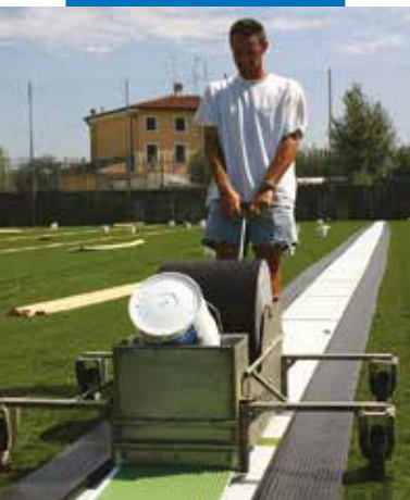
Application of Ultrabond Turf 2 Stars Pro using a continuous and controlled spreading system
