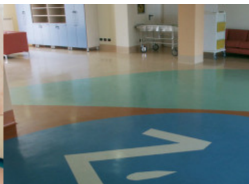
Example of PVC laid in a long-stay ward - San Martino Rest Home - Italy
