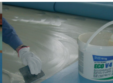
Application of Ultrabond Eco V4SP - San Martino Rest Home - Italy
