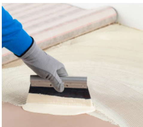
Ultrabond Eco TX2 application
