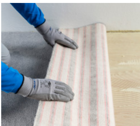
Broadloom carpet installation
