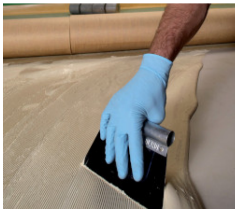
Applying Ultrabond Eco 520
