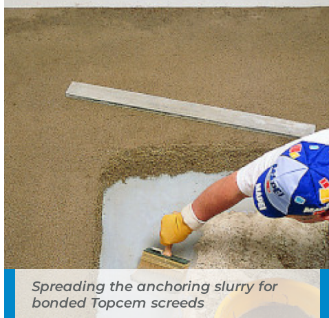
Preparing a levelling strip
