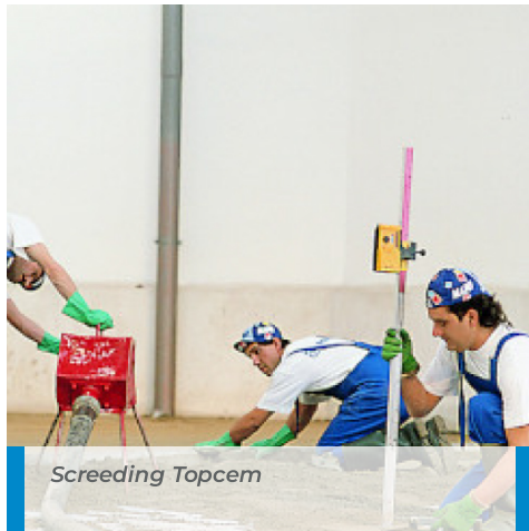
Mixing Topcem with an automatic pumping unit
