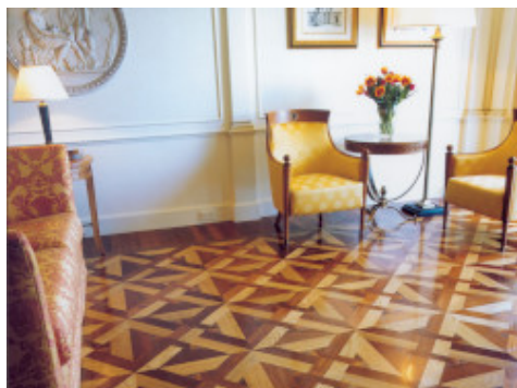
An example of an installation of a wooden floor with Lignobond - Palazzo Versace Hotel - Gold Coast - Queensland (Australia)
