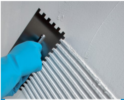
Spreading white Fix & Grout Brick diagonally with a No. 10 notched trowel
