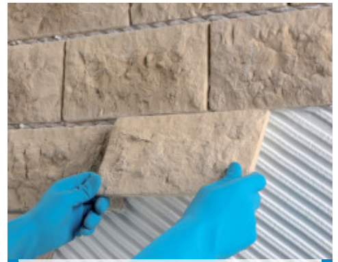
An example of laying ornamental lightweight cementitious composite slips externally
