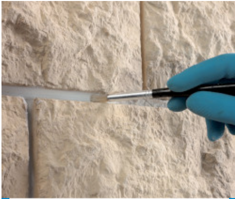
Smoothing the joints with a damp brush
