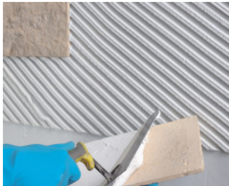
Spreading adhesive on the back of ornamental units
