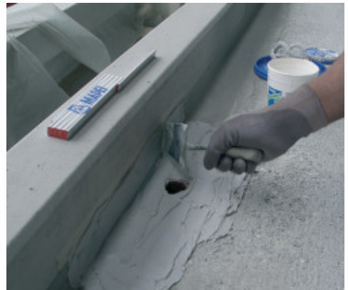
Final covering with Adesilex PG4
