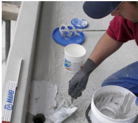
Applying Adesilex PG4 with a trowel
