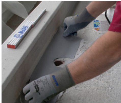
Laying flexible hyphalon brace
