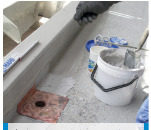
Laying a copper neck-flange and drain spout
