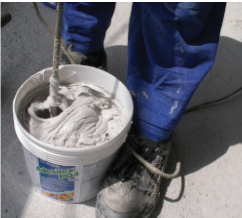
Preparing the mix
