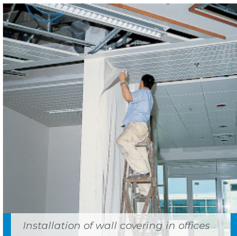
Installing sheets of wall coverings with Adesilex MT32
