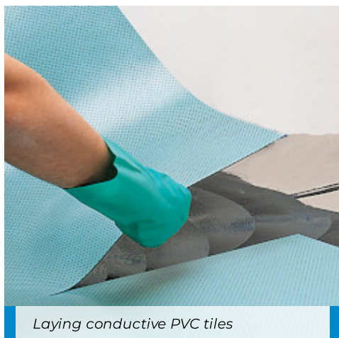
Installing industrial flooring in an electronics company
