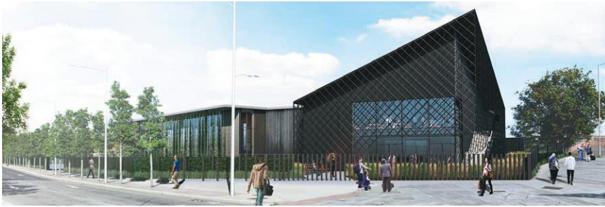
Curious completed on a 1.6 acre site in Ashford for the development of the Curious Brewery.
