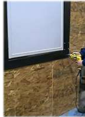
Drill Through Both Angle Edges to Fasten Gate to Threshold.
