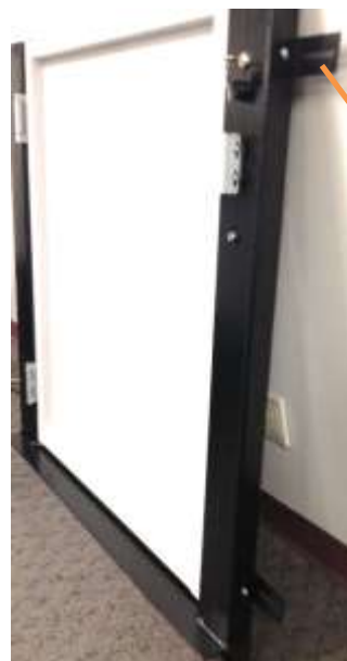
Use Adhesive to Fasten Gate to Existing Structure.
