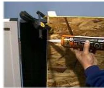
Use Adhesive to Fasten Gate to Existing Structure.
