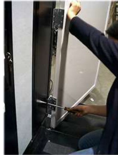
Mount the Carriage Gate.
