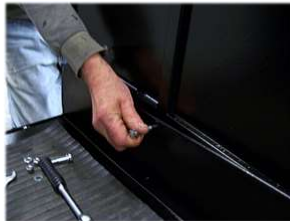
Bolt Handrail to Platform.
