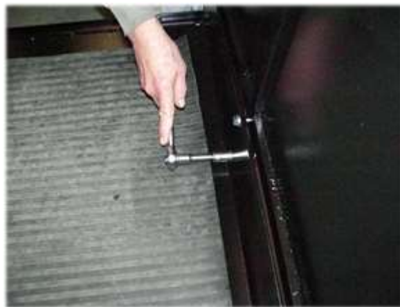
Bolt Handrail to Platform.
