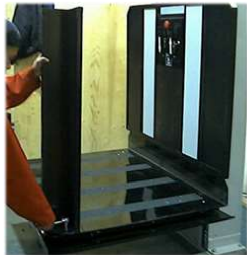
For Adjacent Unit, Mount Corner Post
