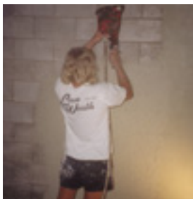
1.1 Application of Astec Waterproof Render
