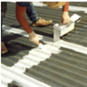
1.1 Sontara used for seam sealing sheet joins in a metal roof
