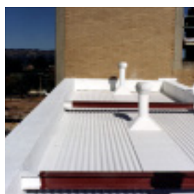
1.2 It will prevent underfilm corrosion of fresh paint work
