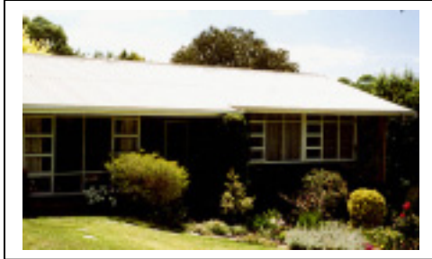
Standard White S.R.I. 100.11 Surface Temp at 37°C = 45°C
