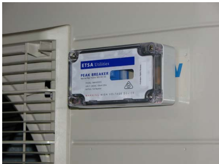
Photo: “Peak Breaker” Fitted Externally To The Compressor
