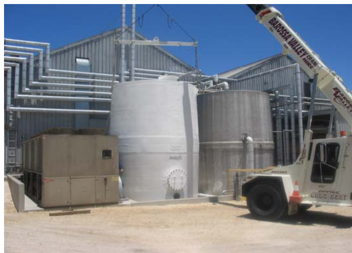
Photo: 45,000 Litre Insulated Tank at St Hallett Wines
