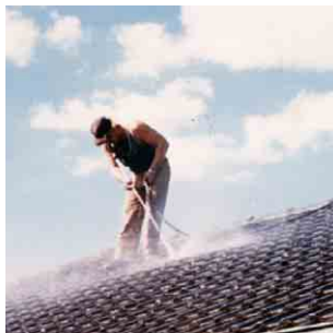
1.2 High pressure water cleaning
