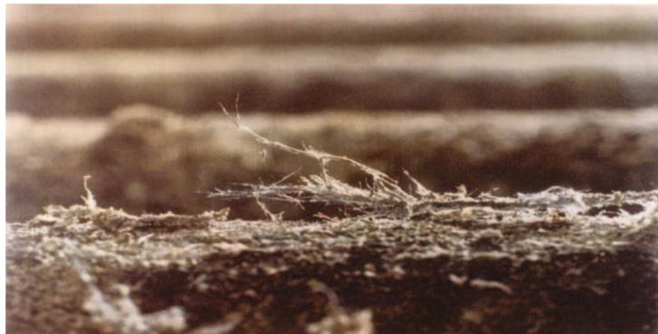
Over the years asbestos cement roofs deteriorate through weathering. The surface layer of cement decays, exposing the underlying asbestos fibers to the environment through an ongoing process of erosion. As a result, the asbestos cement thins, becomes brittle and the structural stability of the roof is greatly reduced. The material becomes dark, increasing the internal temperature of the roof cavity and lichen growth detracts from the aesthetics of the building.
