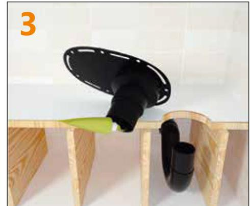
Connect the drain to the P-trap. Glue coupling reducer (if necessary) to the drain body first, then to the P-trap. Apply glue to both ends for a safe installation.
