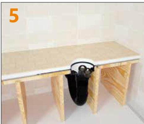
Do not obstruct the hole of the drain body. Be sure to leave enough space around the drain body.
