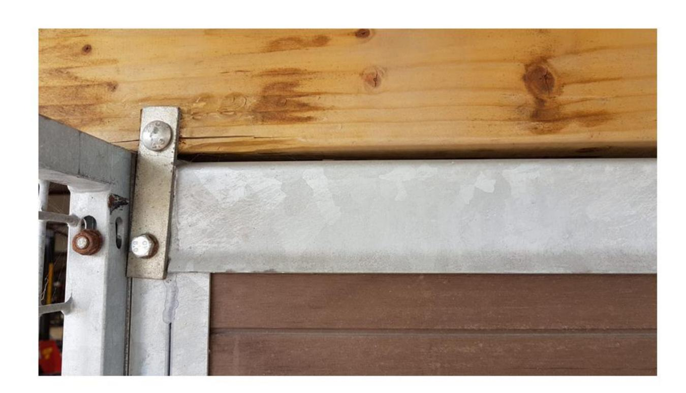
Once all the roof brackets are secured like above it is now time to attach the timbers. The larger 6x2 timber goes at the front and the sm aller 3x2 timber goes at the rear.
