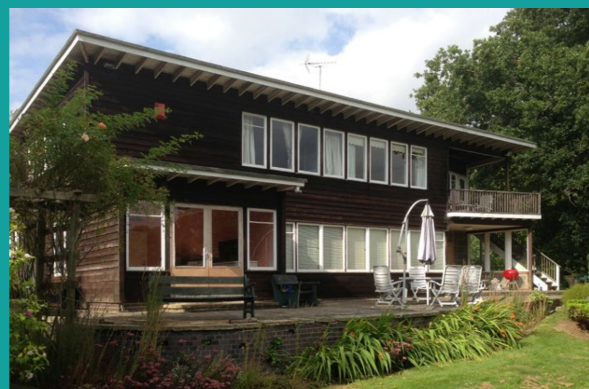
The Wood House, Shipbourne, Kent, 1937
