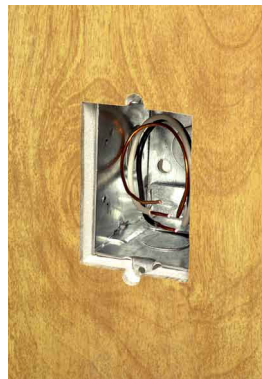
Electrical box is behind the new finished wall surface.
