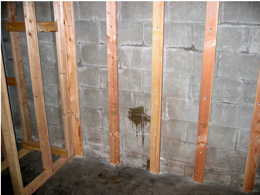
2 x 4 furring strips fastened to concrete block with concrete screws.
