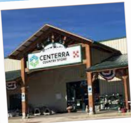
Centerra Country Store 1290 Middle Rowsburg Road Ashland, OH 44287
