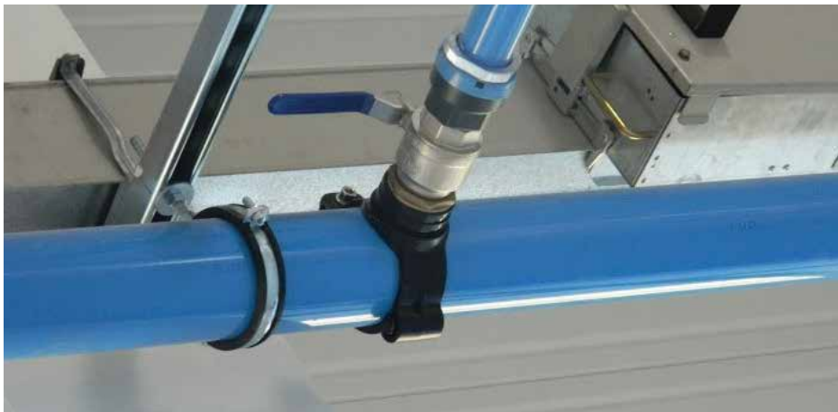
Typical Application for Saddle Branch
