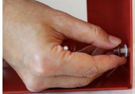
The flat washer limits side-to-side movement of the letter box. It is used if there is no paint on the edge of the pivot pin near the housing.
