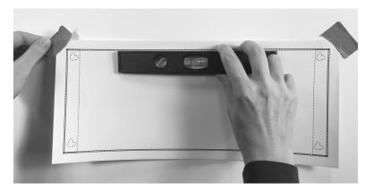
**Siding Not Flat**: you may need to move the Plaque up or down so that it makes contact with the wall where the four screws will enter the wall. Shims may be required on either the top two or bottom two mounting locations. In the alternative, the plaque can be mounted using only the top two holes.
