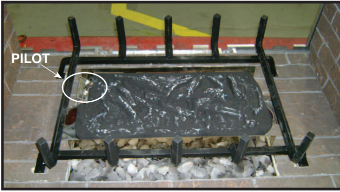
Figure 2. Burner and grate from front.
