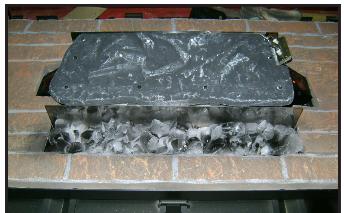
Figure 11.16 Finished Ember Bed
