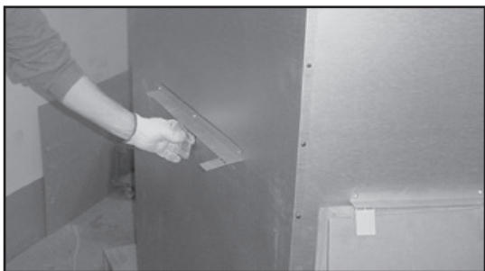
Figure 3.7 Bend Refractory Brackets Back Down
