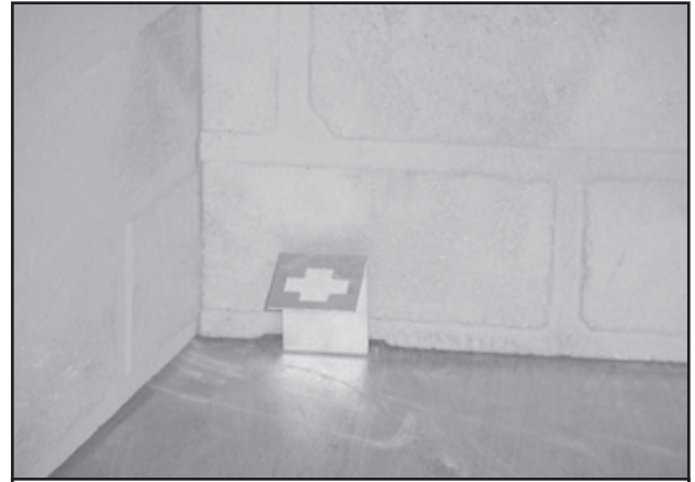
Figure 8.8 Grate Retaining Bracket in Place
