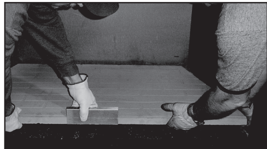
Figure 3.10 Lifting Out Hearth Stone
