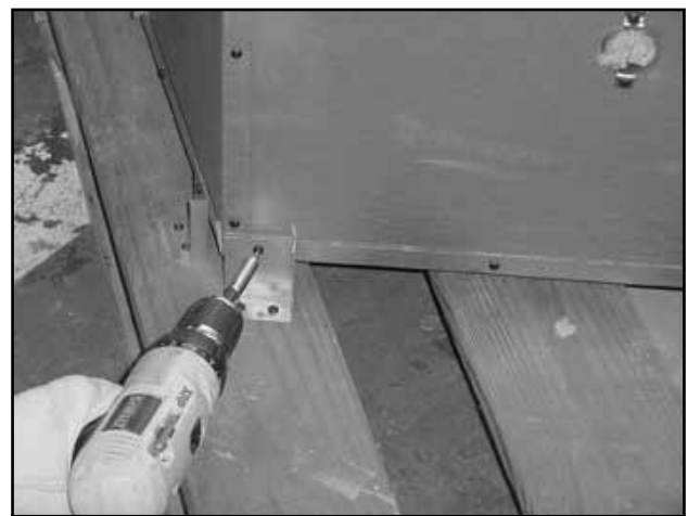
Figure 3.11 Removing Shipping Brackets
