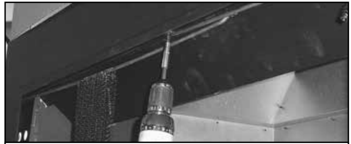
Figure 3.8 Removing the Screen Rods
