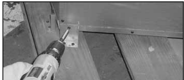
Figure 3.10 Removing Shipping Brackets
