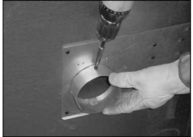
Figure 3.18 Attaching Outside Air Kit Collar
