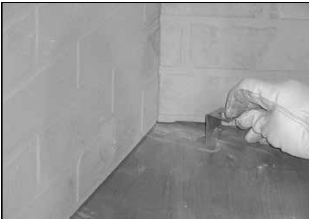
Figure 8.7 Slide Grate Retaining Bracket into Notch
