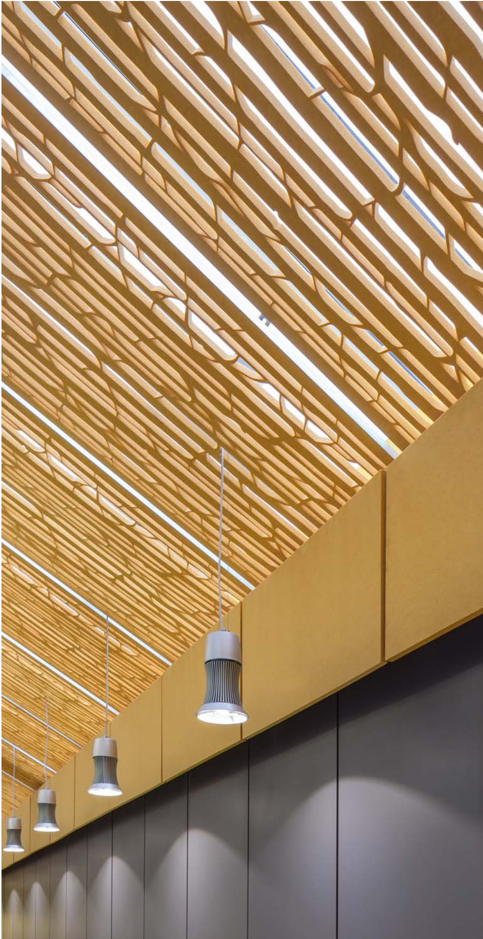
● Custom Cascade Static Screens in Senado
