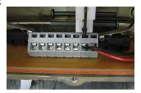
1. Take a small flat blade screw driver and insert it into the slot above where you want the wire to go.
