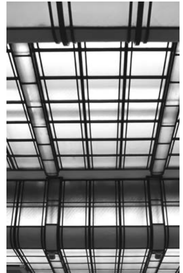
8. Inter-war Kaunas was built using traditional methods and traditional materials: wood and brick. The interiors of public buildings, however, also revealed a bold use of new glass and concrete construction. Shown here is the lobby ceiling of the Lithuanian State Savings Bank (today the Kaunas City Municipal Building) in 1940. Photo: Vaidas Petrulis, 2012
