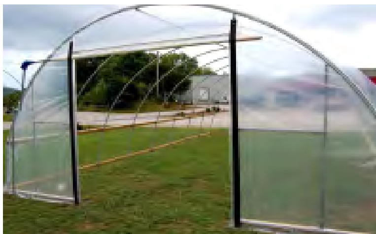
Finished Roll Up Door
