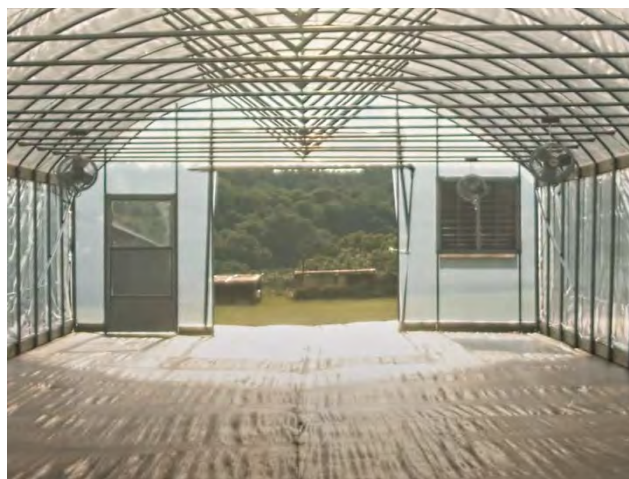
Finished Roll Up Door
