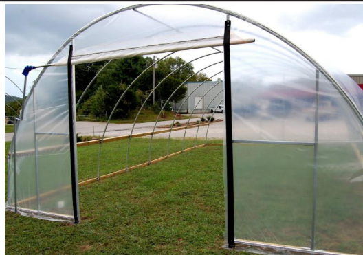
Finished Roll Up Door
