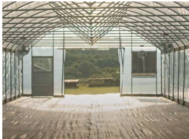
Finished Roll Up Door
