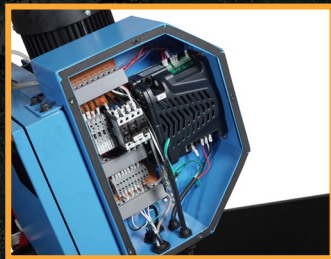
AN INVERTER ALLOWS THIS SAW TO RUN ON 115V SINGLE PHASE POWER DRIVEN BY A DURABLE THREE PHASE MOTOR
