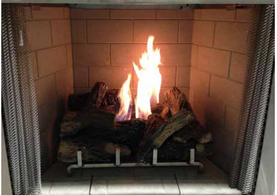
Figure 23 - Proper Burner Flame Appearance
