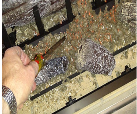
Figure 9- Adjusting of Flame Pattern
